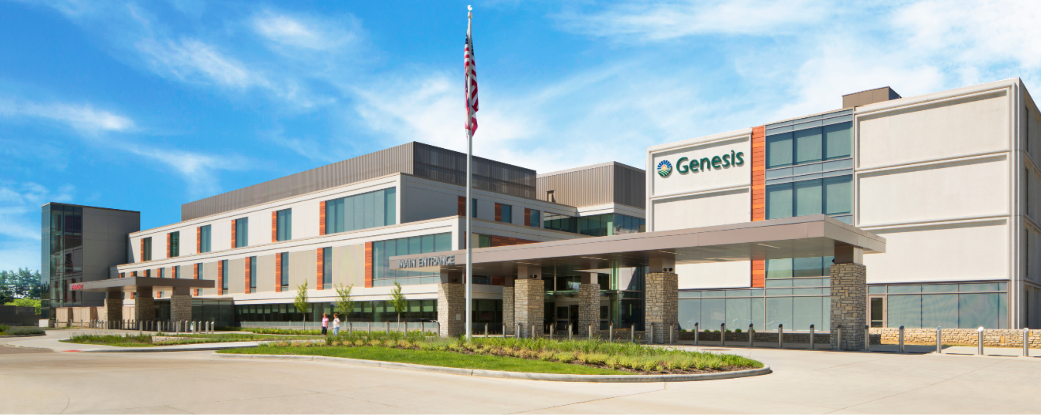
Exterior details - Terra cotta tiles, textured precast, and fritted glass
