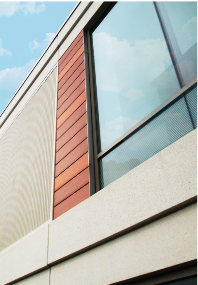
Exterior details - Terra cotta tiles, textured precast, and fritted glass
