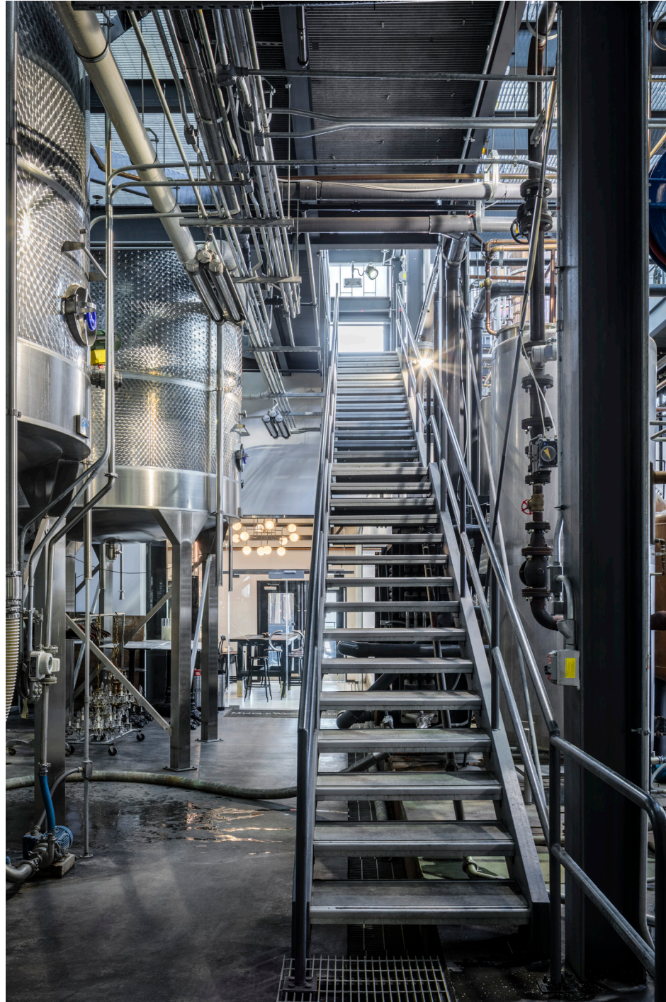
Access to Mezzanine
